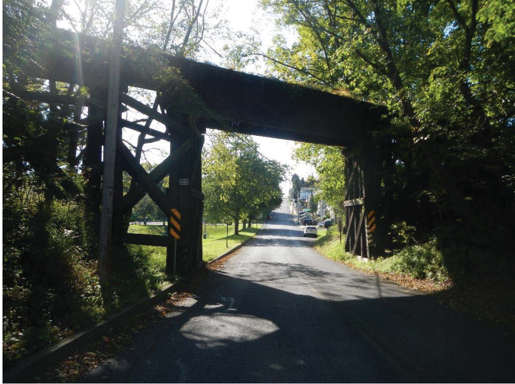
5. Partial Left (North) Elevation View
