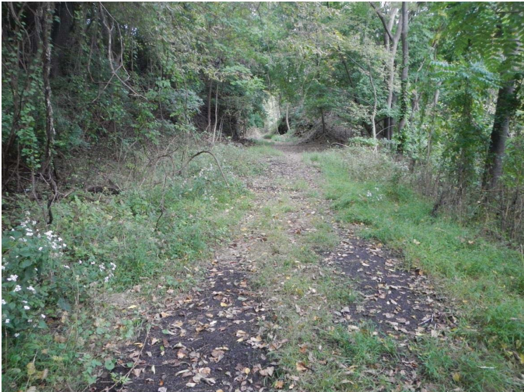
4. View of Far (East) Approach Looking East
