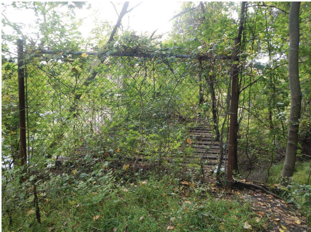
2. View Over Structure From Far (East) End
