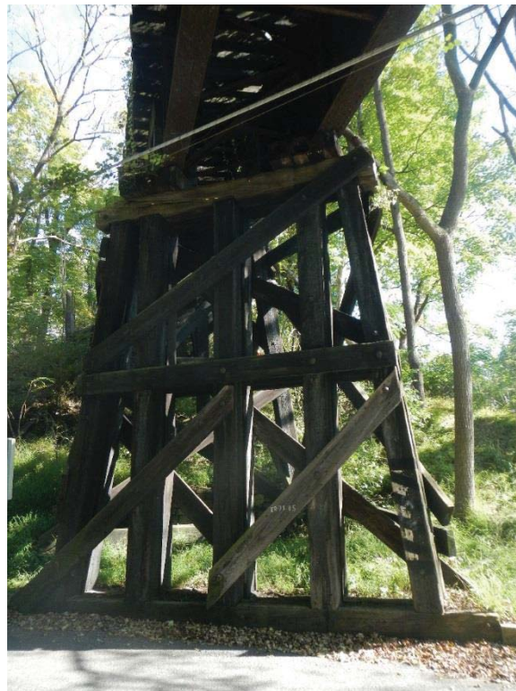
10. Pier 5 Near (West) Elevation (Typical Main Span Pier)
