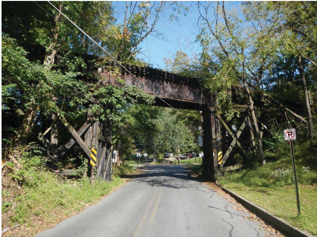
6. Partial Right (South) Elevation View
