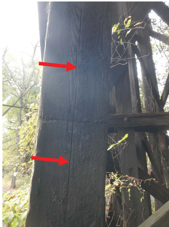
52. Pier 12 Column 4 Split Far (East) Face
