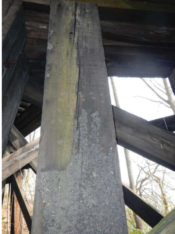
41. Pier 5 Column 2 Split Near (West) Face
