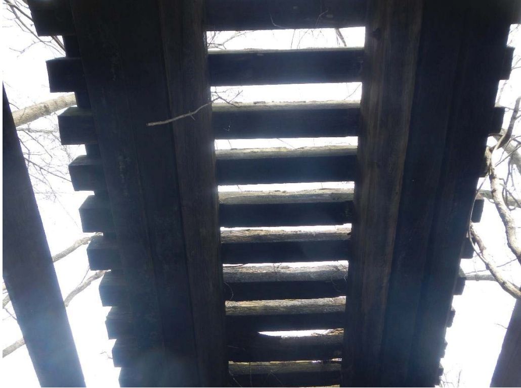
7. Span 2 Superstructure (Typical Approach Span Superstructure)
