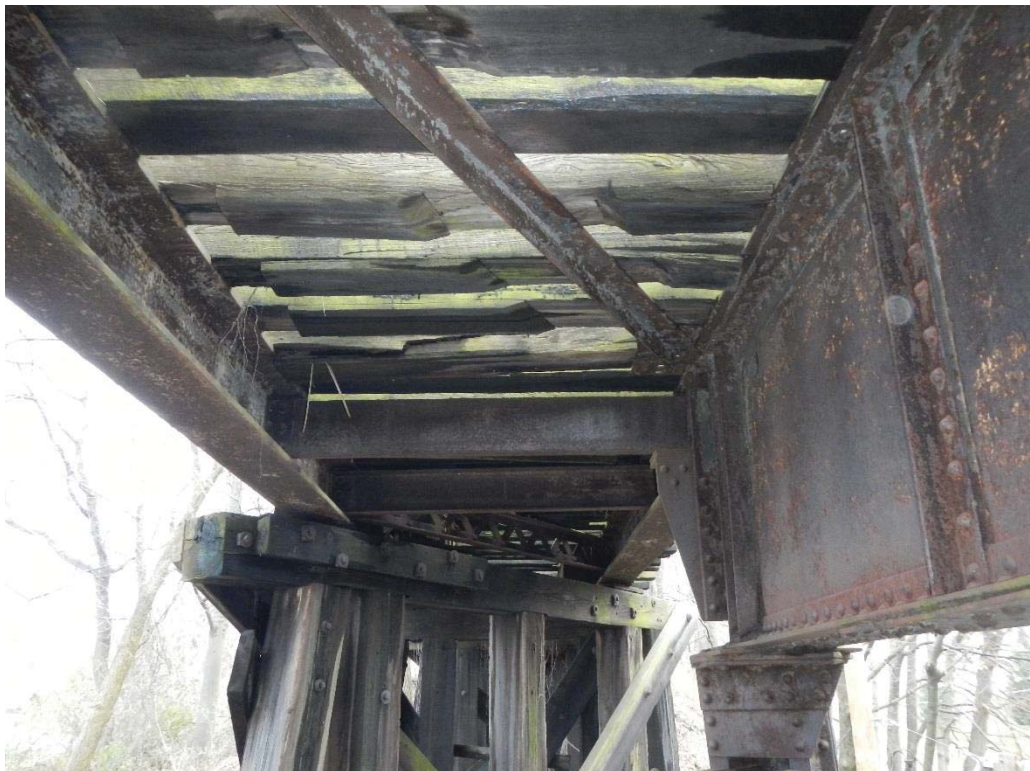
8. Span 7 Superstructure (Typical Steel Approach Span Superstructure)
