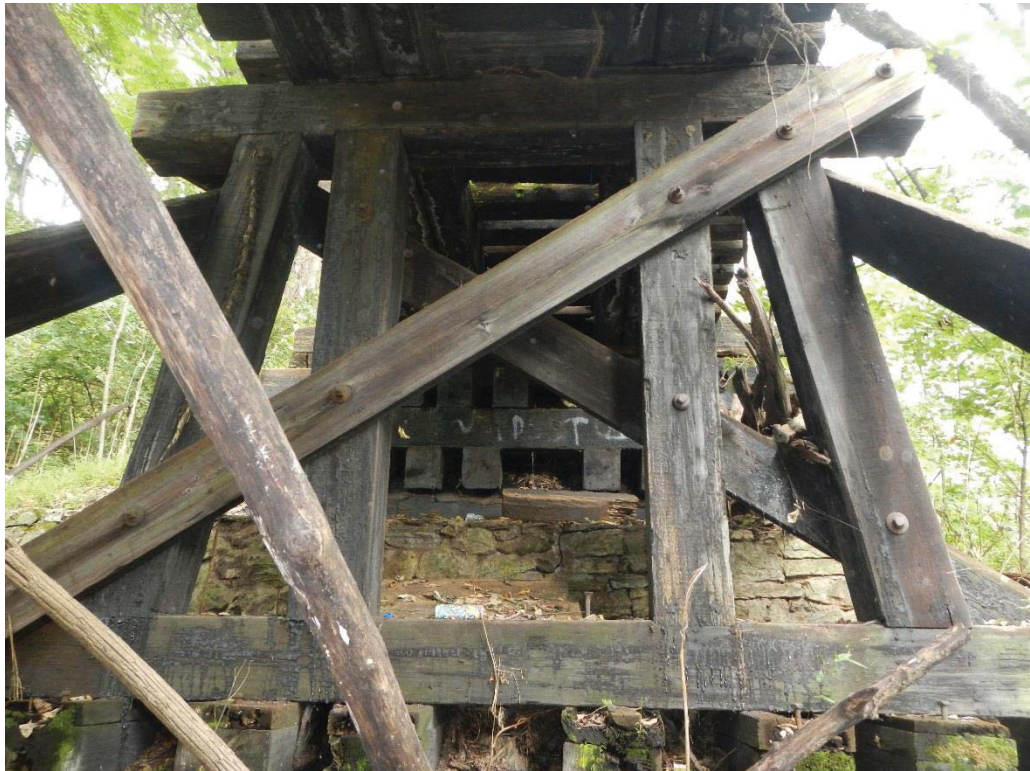
10. Pier 18 Near (West) Elevation (Typical Approach Span Piers)
