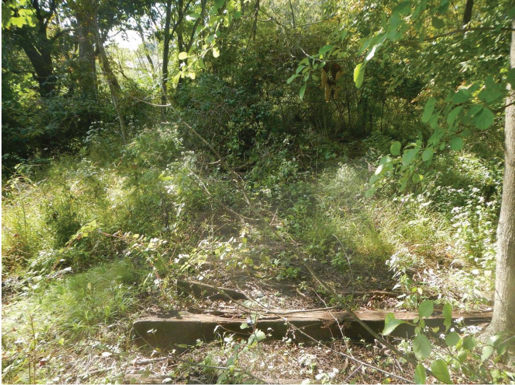
3. View of Near (West) Approach Looking West
