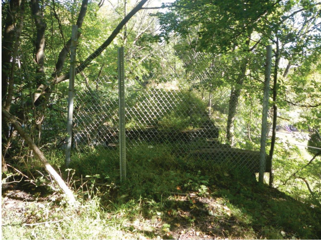
1. View Over Structure From Near (West) End
