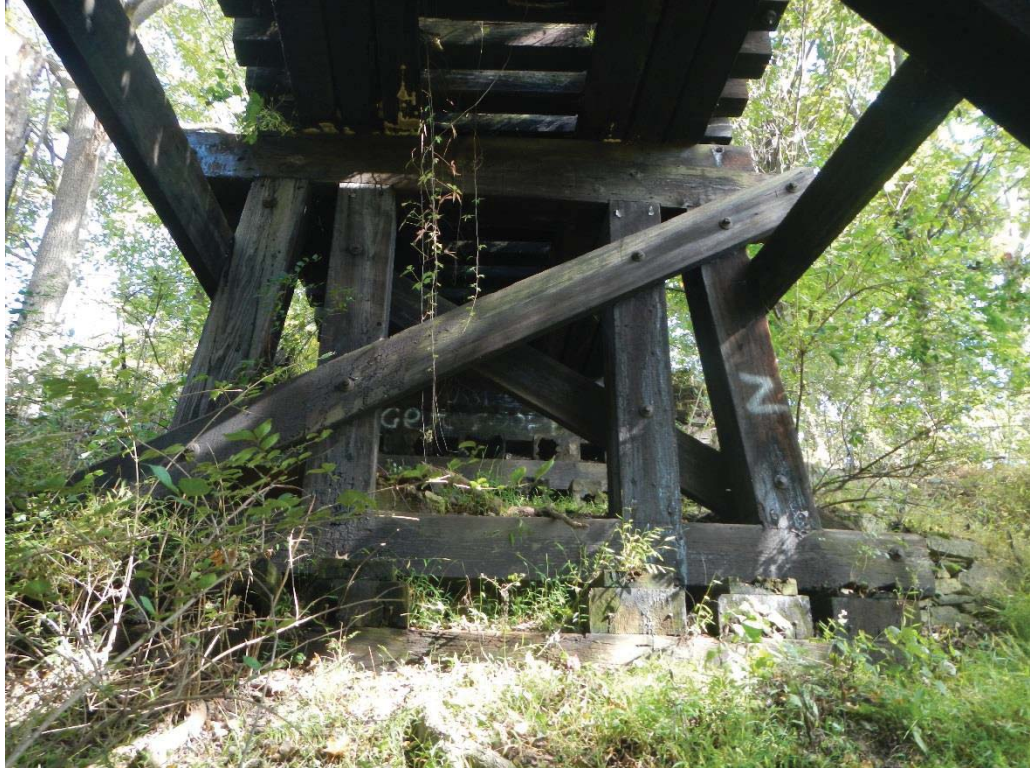
9. Pier 8 Near (West) Elevation (Typical Approach Span Pier)
