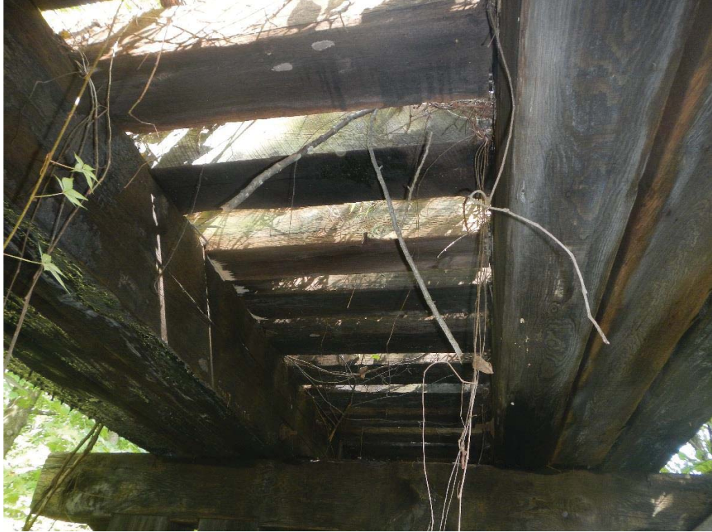
7. Span 2 Superstructure (Typical Timber Approach Span Superstructure)
